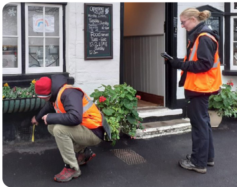
Property survey for flood resilience measures.
