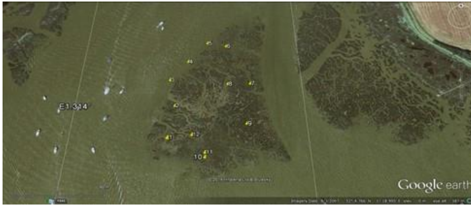
Figure A1. Google earth aerial image showing location of posts on Loder's Cut island (plotted from co-ordinates obtained by River Deben Association).
