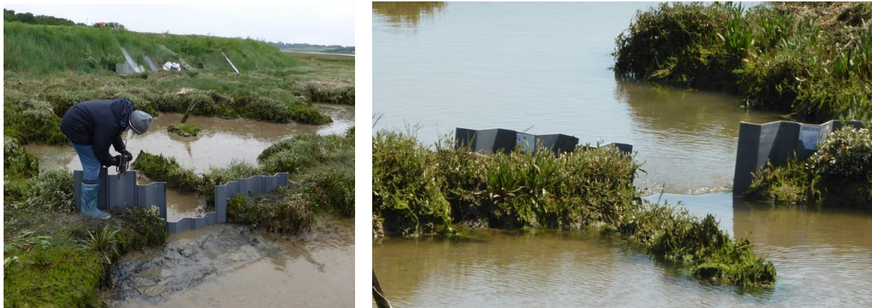
a) Installing the sheet piling
