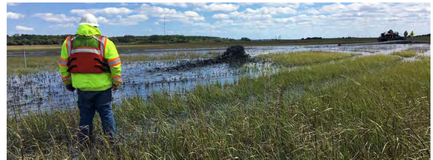
Monitoring dredged sediment placement as part of a 2 ha thin layer placement project at Jekyll Creek, USA (Clay McCoy, USACE Jacksonville District).
