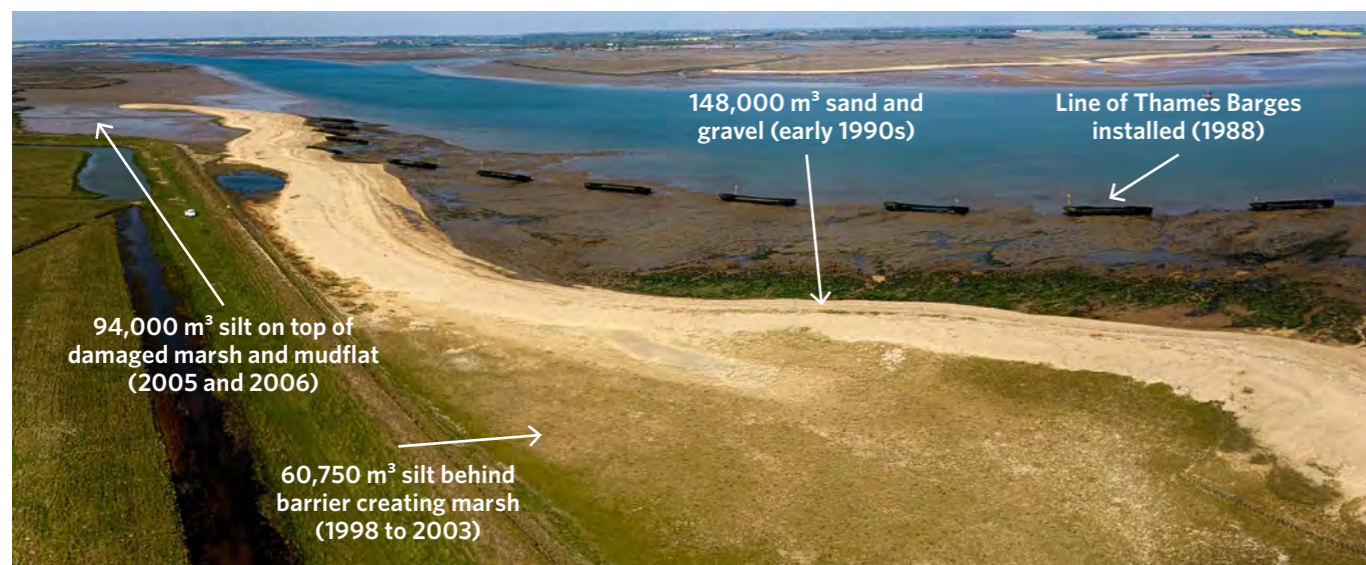
Horsey Island, Essex, showing some of the range in volumes, particle sizes and locations of beneficial use campaigns, and other works, undertaken here over the last 30 years (Image: Jim Pullen Surveys).
