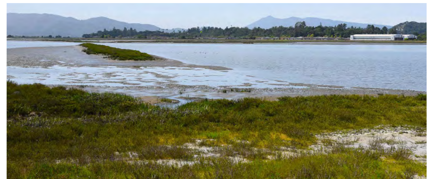
Approximately 4.5 million m 3 of dredged material was used to raise marsh levels and created vegetated berms that provide a seed source, disrupt fetch, reduce wave heights and encourage further deposition across the Hamilton Wetlands, USA (USACE San Francisco District).
